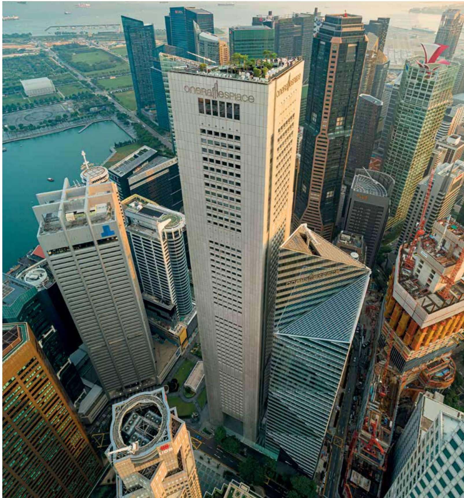
One Raffles Place Towers 1 and 2 are certified Green Mark Gold and Platinum respectively by the Building and Construction Authority of Singapore
