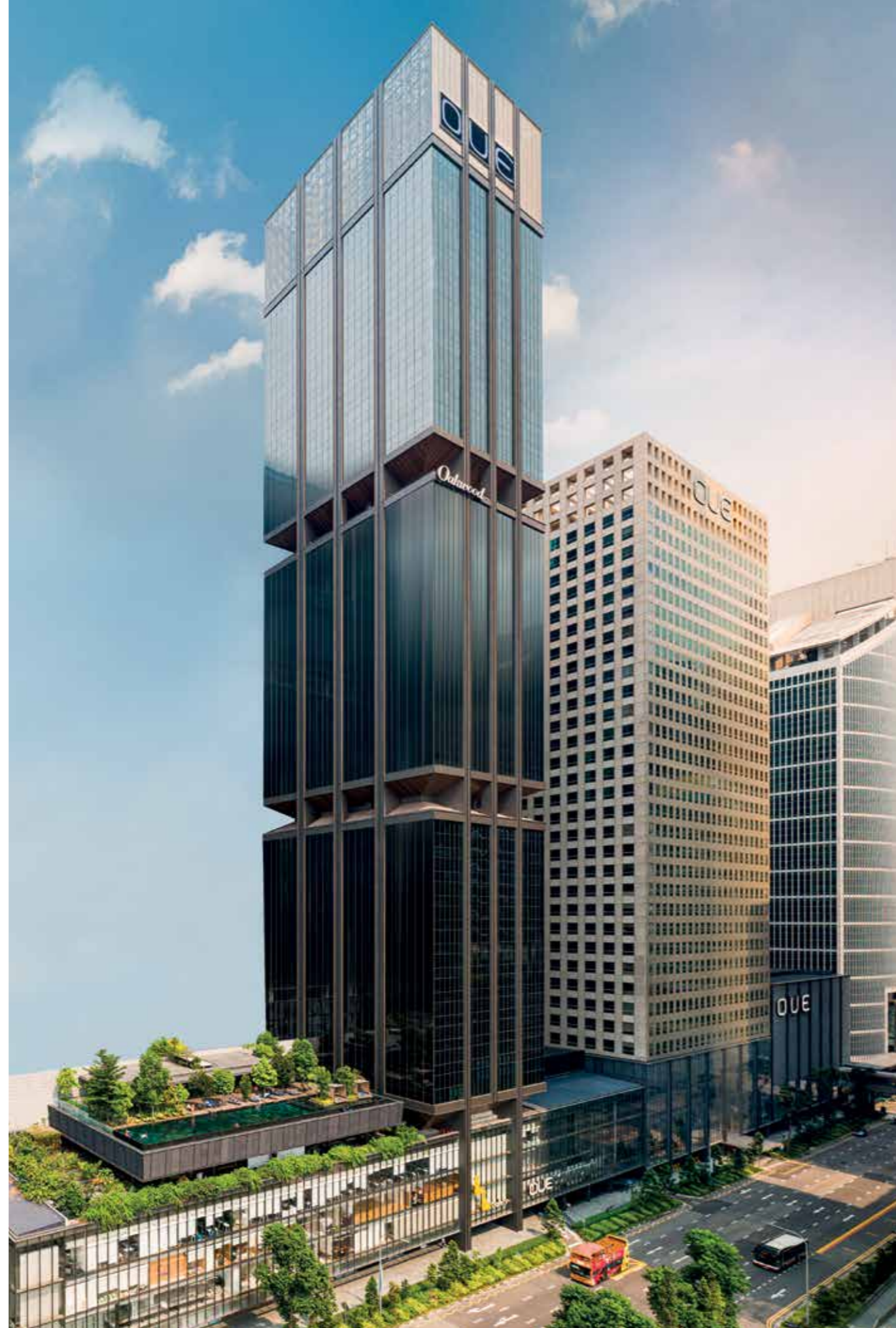
OUE Downtown Office towers rise above the development's integrated six-storey retail mall
