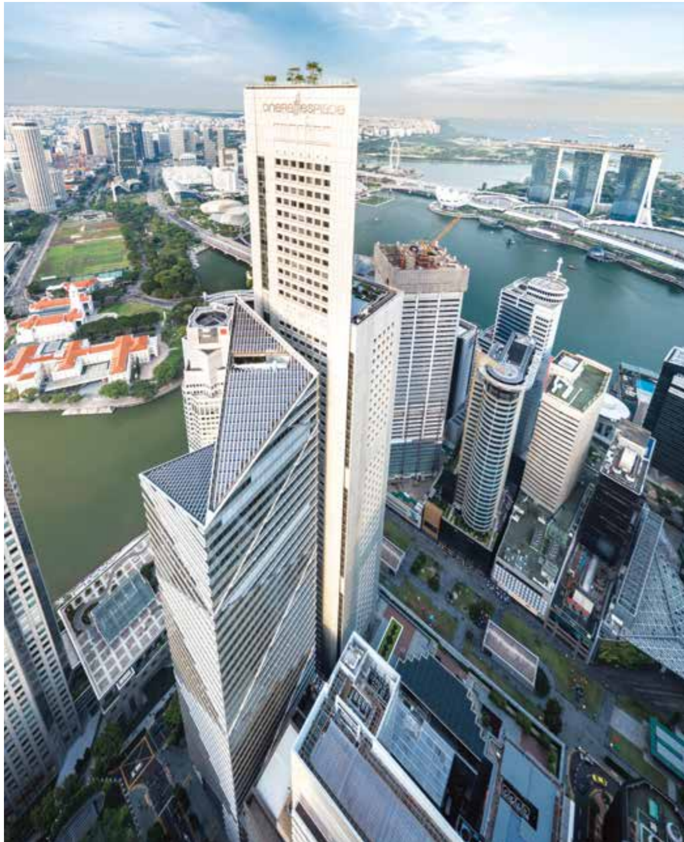
One Raffles Place Towers 1 and 2 – the height of distinction on the CBD skyline
