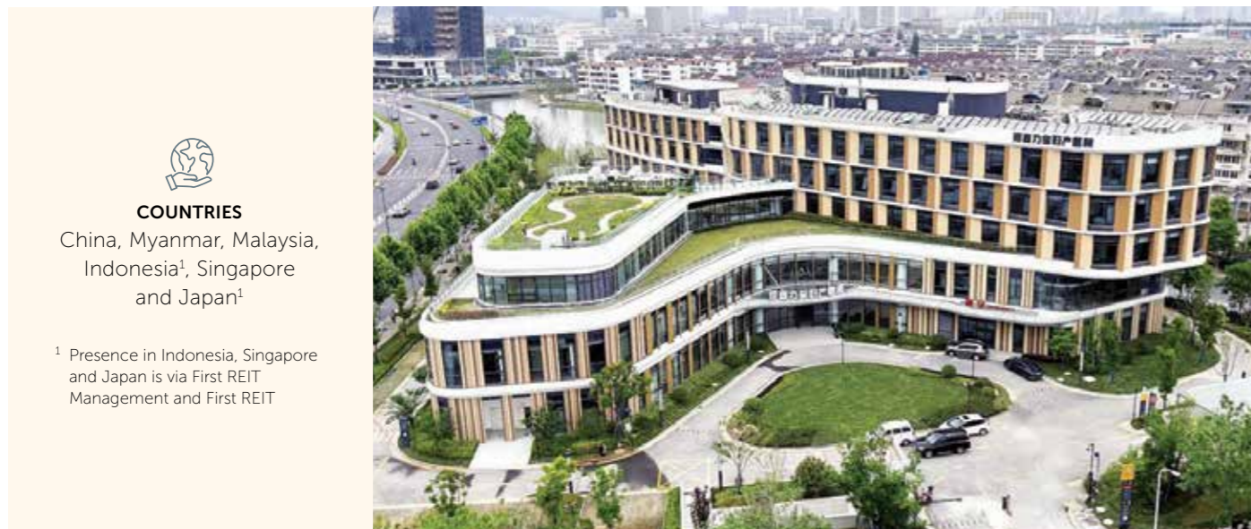
Changshu China Merchants-Lippo Obstetrics & Gynaecology Hospital – positioned to cater to an affluent market segment
